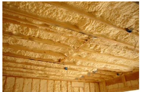
This polyisocyanurate foam insulation must have an approved thermal barrier between it and the living space.
