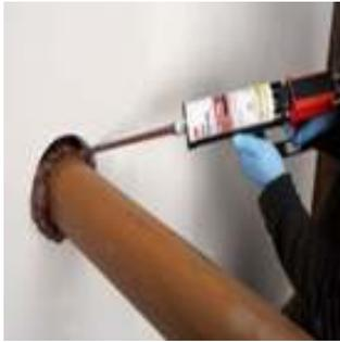
3M Fire Protection Products introduces 3M FIP 1-Step Firestop Foam, a breakthrough technology that is UL tested and listed and satisfies the International Building Code for passive fire protection. 3M FIP 1-Step gives contractors an outstanding alternative to mineral wool, bricks and runny, ineffective foams, and enables firestop installations to be completed up to three times faster than traditional methods.
